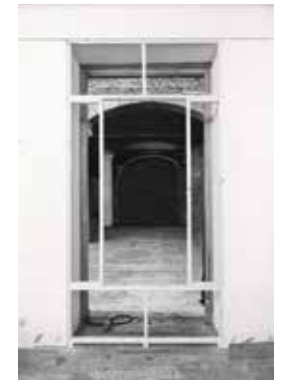
a framework is installed ...
