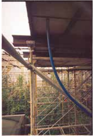
Snaking soil pipe.
