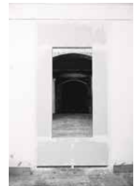
and four plaster boards seal the doorway.
